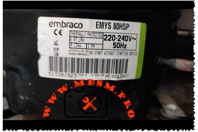
EMYS80HSP is a refrigerator compressor model made by Embraco, a company known for manufacturing reliable and energy-efficient compressors. Here's a breakdown of the code:
