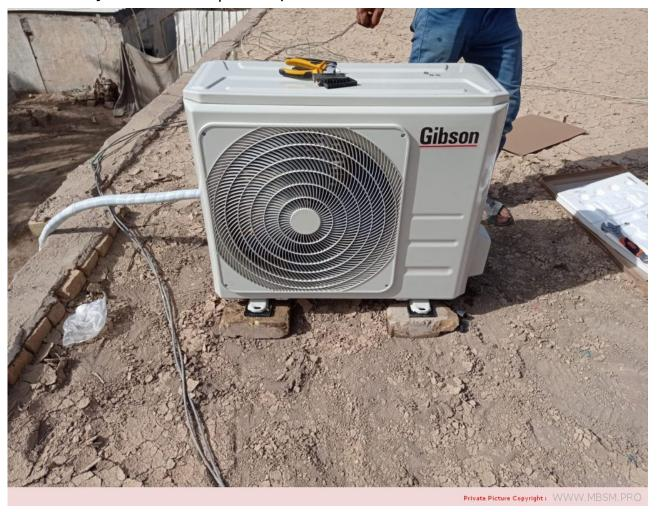
Mbsm.pro, air conditioner, GiBson, GS18K11BCHI, 18000 btu, 15 A, 2900 w, Cooling, Heating, r410a, 1400 G, 220v50hz, T1
