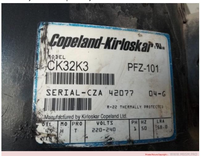
Mbsm.pro, Compressor, CR-32K3, CK-32, PFZ-101, Copeland, air conditionnel, r22, 32000 btu
