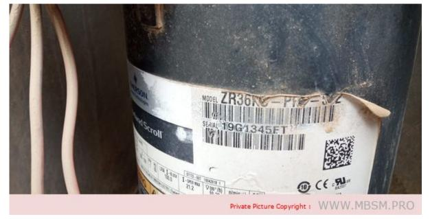
Mbsm.pro, 30000 BTU, Copeland, Scroll, Compressor, ZR36KC-PFJ-522, 3 Ton, r22,
