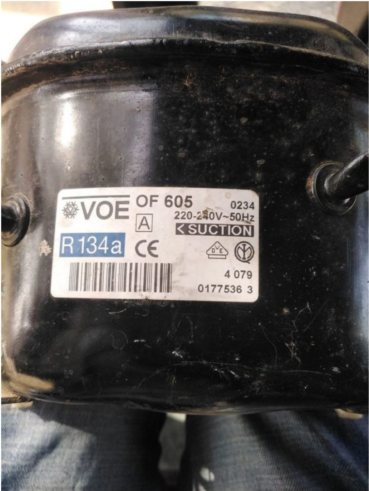
ZANUSSI FRIDGE, FREEZER COMPRESSOR, OF605, R 134a, 1/9 HP, LBP, 50w
