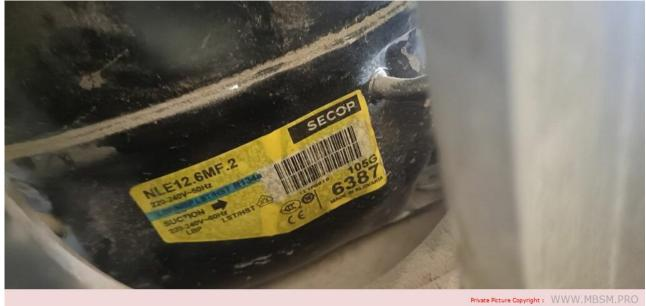
Mbsm.pro, Compressor, NLE12.6MF.2, SECOP, 105G6387, DANFOSS, R134a, 1/2 Hp, lbp
