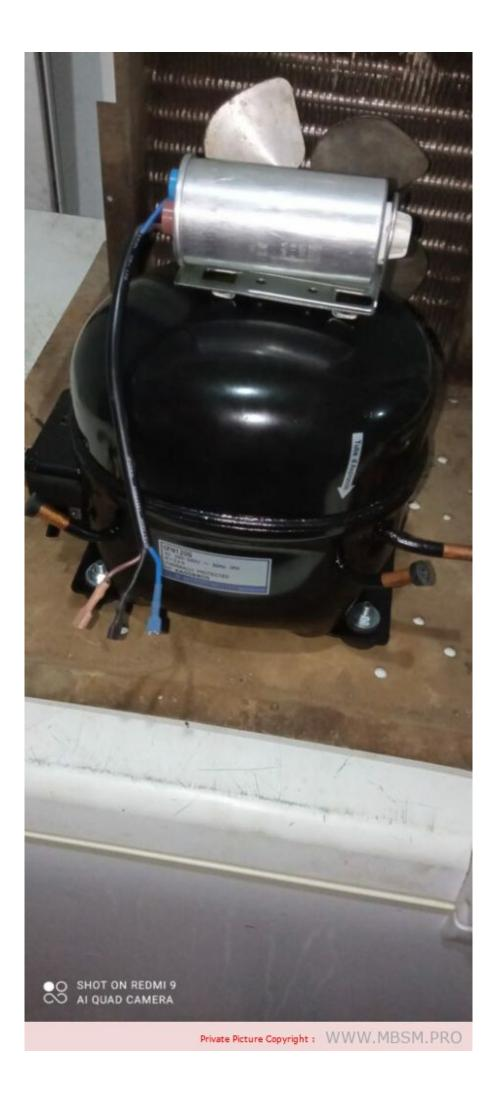
Mbsm.pro, Compressor, Gold, cfn120g , Capacitor 64  $\mu F$
