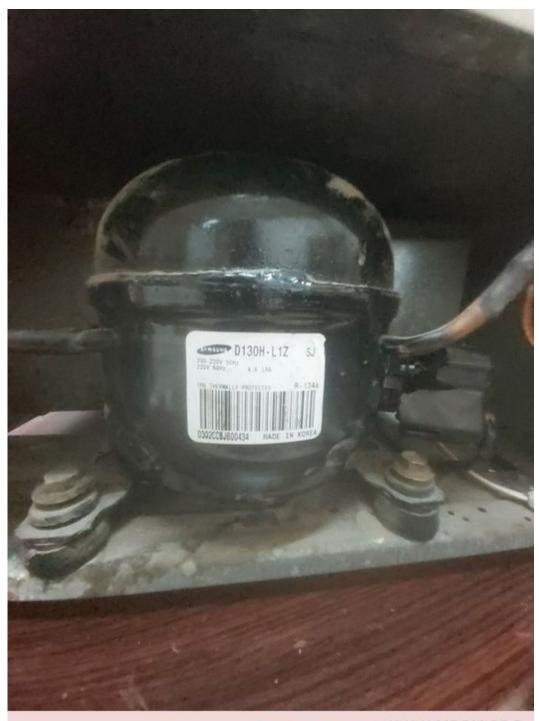
Private Picture Copyright: WWW.MBSM.PRO Refrigeration, Compressor, 1/10 HP, R-134A, Samsung, CD130C-L1Z2
