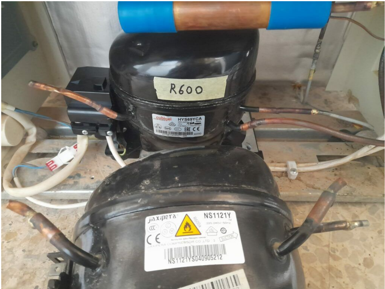
Mbsm.pro, Jiaxipera, NS1121Y, 1/4 hp++, 1/3 hp-, 214Kcal, R600a, 220V
