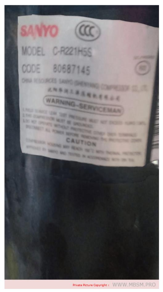
Mbsm.pro, compressor, Sanyo, Rotary, Split system air conditioner, Compressors, C-R221H5S, S6231526791, 24000 btu,
