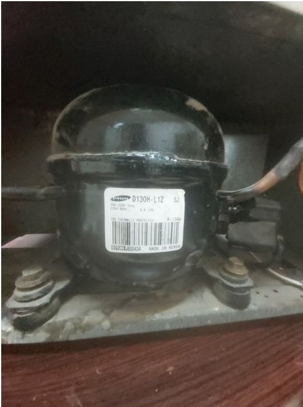
Refrigeration, Compressor, 1/10 HP, R-134A, Samsung, CD130C-L1Z2
