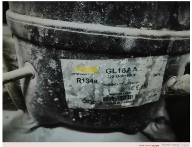
Mbsm.pro, Compressor, coolant, Cubigel, R134a, GL18AA, 220-240V, 50Hz, 3/8 hp++, 1/2HP-
