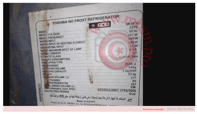
Mbsm.pro, Toshiba, no frost, refrigerator, Gr-ef31
