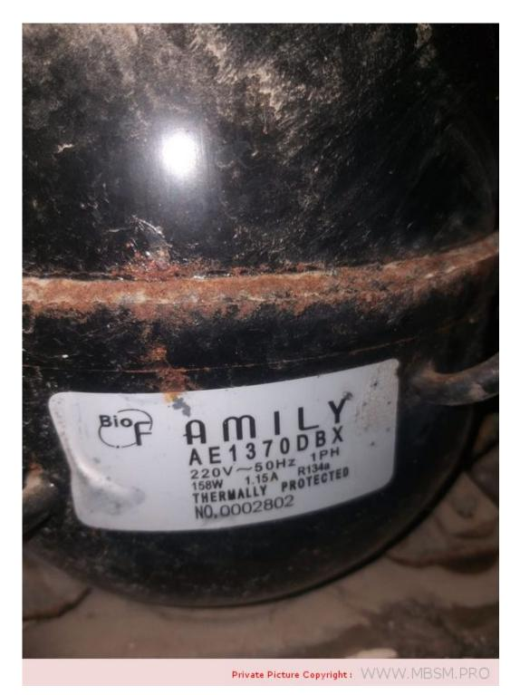
Mbsm.pro, Compressor, AE 1370, AE1370, 1/5 hp ++, 158 w, 1/4 hp—, lbp, R134a, replaced by HYE69YK, raded Amp 1.5 A
