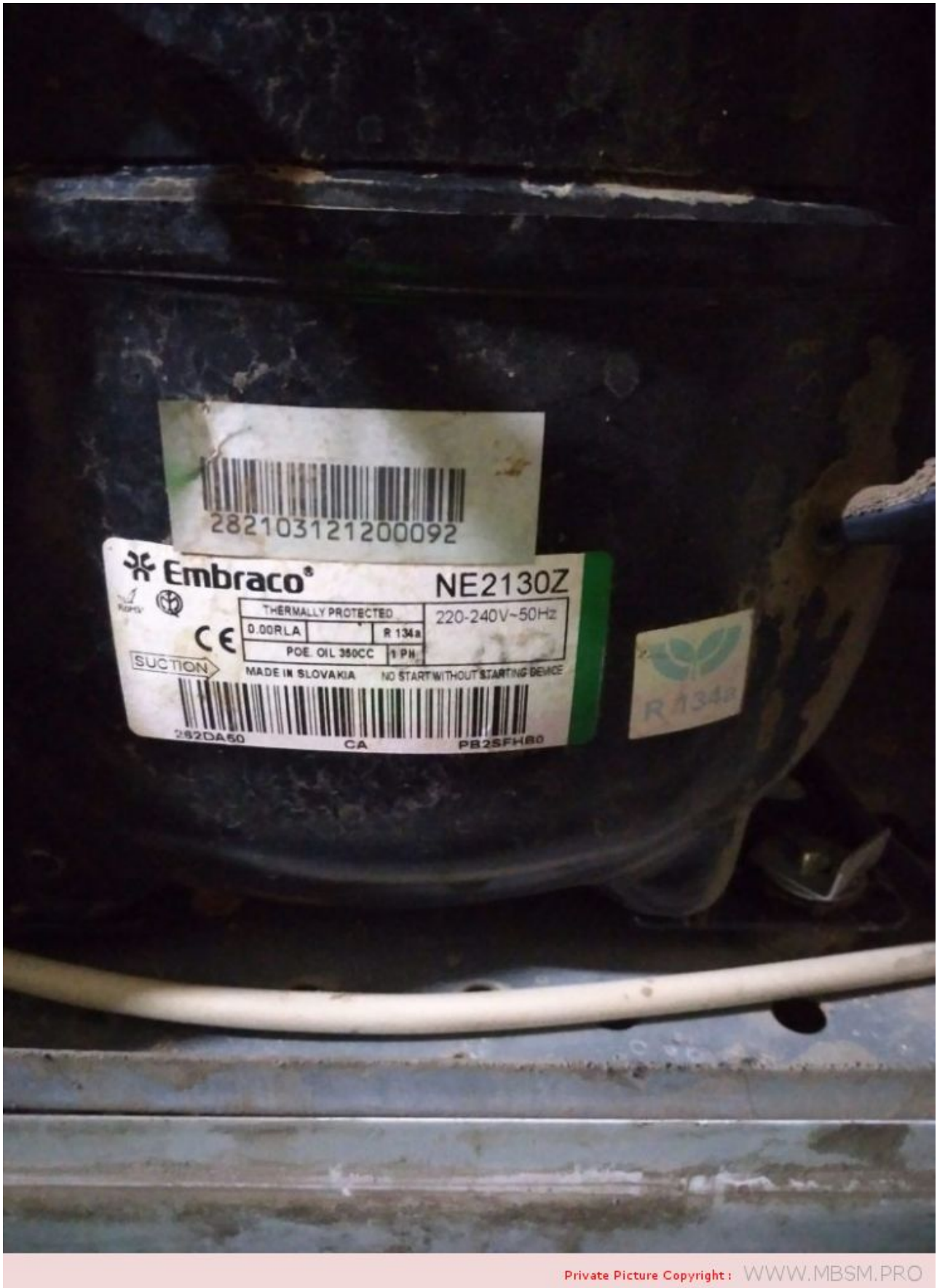
Mbsm.pro, Compressor, NE2130Z, R-134a, 1/3HP, 230V, Embraco, LBP
