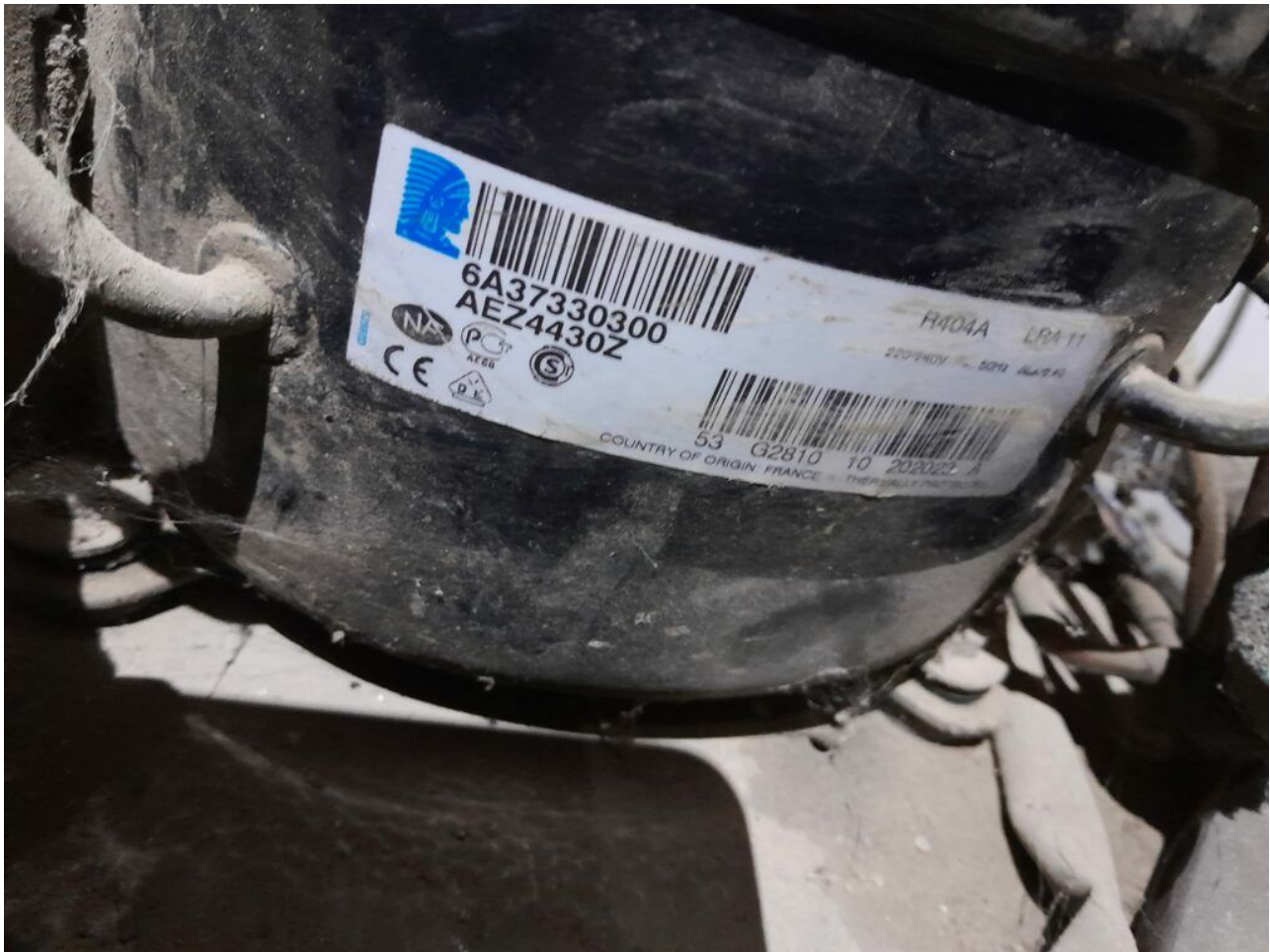
Mbsm.pro, Compressor, AE4430Z, R-404a, 1/4 HP , 230V, hbp
