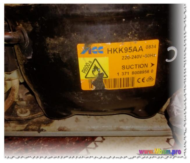
The **Comp HKK95AA** is a compressor designed for refrigeration applications, specifically operating at **220-240V** and **50Hz**, with a capacity of **1/5 HP (167W)** and using **R600a refrigerant**. Here are some key details:
