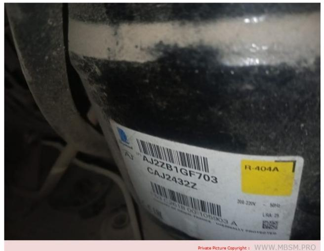
Mbsm.pro, CAJ2432Z, AJE2422ZHZ, 3/4 hp, Tecumseh, Compressor, R404a, Lbp, 480 w,  $18.3\text{CM}^3$
