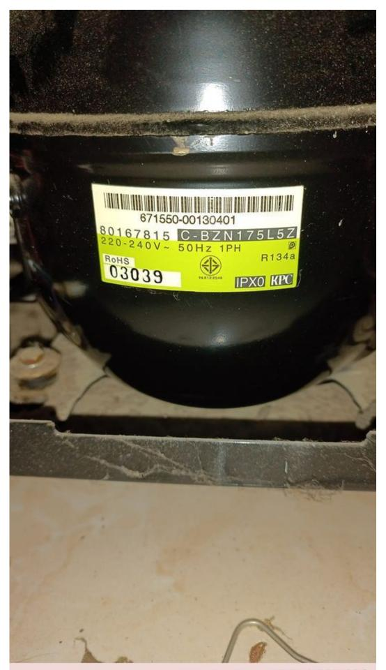
Private Picture Copyright: WWW.MBSM.PRO Mbsm.pro, Compressor, C-BZN175L5Z, KULTHORN, piston, refrigeration compressor, 1/5 hp
