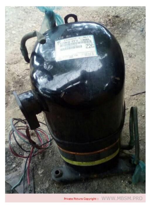
Mbsm.pro, Compressor, Copeland, CI20KQ-PFV, 240v/ 230/PH1/60hz , 1.5 hp, R-22 , 18,300, A/C
