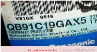
Mbsm.pro , Qb91c19gax5 , Panasonic , Compressor cooling , 1/3HP , 236W , 1Ph , 220V
