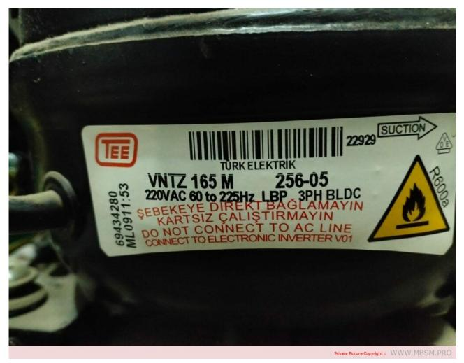
Mbsm.pro, Beko, Tee, Compressor, Turk, VNTZ165M, VNTZ 165 M, VNTZ165MT / VNTZ165M, R600A, lbp, Inverter, variable speed, blcd, 165 kcal, 195 w
