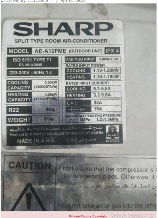
Mbsm.pro, Air conditioner, Sharp, AE-al2fme, 12000 btu, r22, 860 g, 1.5 hp, 1 ton, cooling, heating, T1, PH 1
