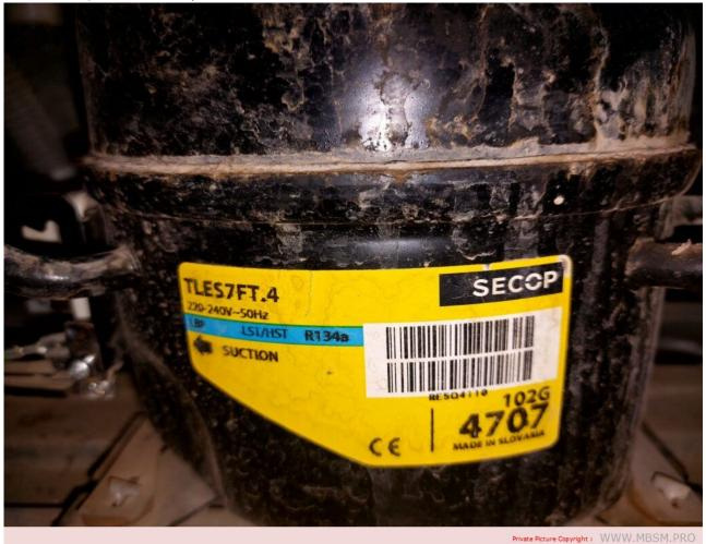
www.mbsm.pro , TLES7FT.4 , COMPRESSORE SECOP ,TLES7FT.4 , R134a , LBP ,Danfoss compressors ,medium temperature, HMBP
