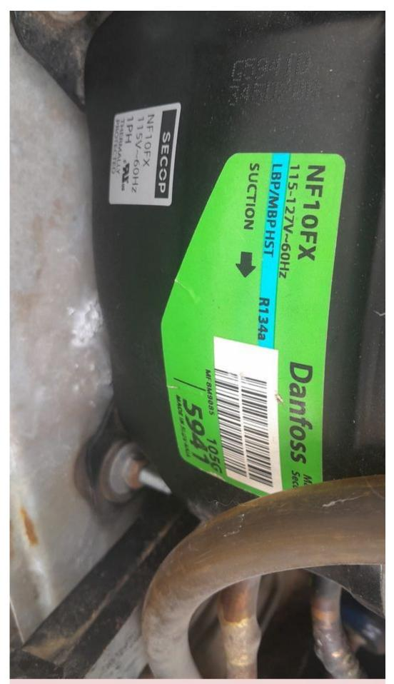
Private Picture Copyright: WWW.MBSM.PRO Mbsm.pro, Compressor, nf10fx, Danfoss, 1/3 hp, LBP, MBP, 1046 btu, 115 v
