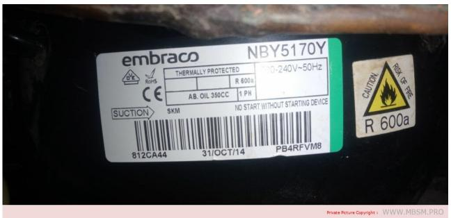
With a cooling capacity of 842 W and robust construction, the NBY5170Y is ideal for commercial refrigeration, air conditioning, and heat pump systems
