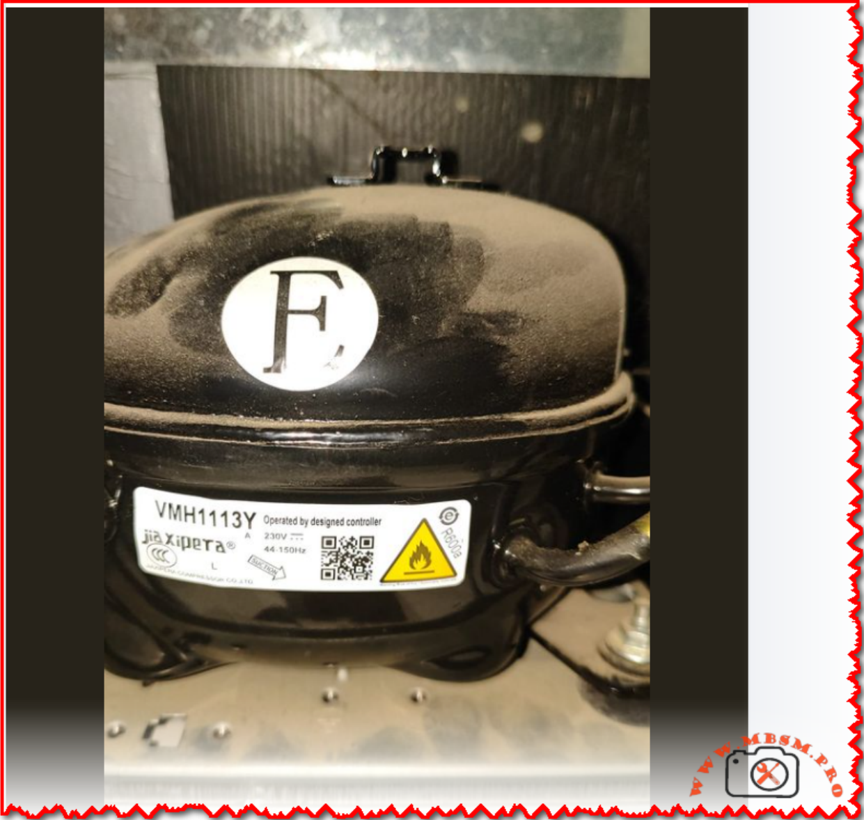
Mbsm.pro, Inverter, BLCD, compressor, refrigerator, R600a, JIAXIPERA, VMH113Y, 1/6 hp, r600a, lbp
