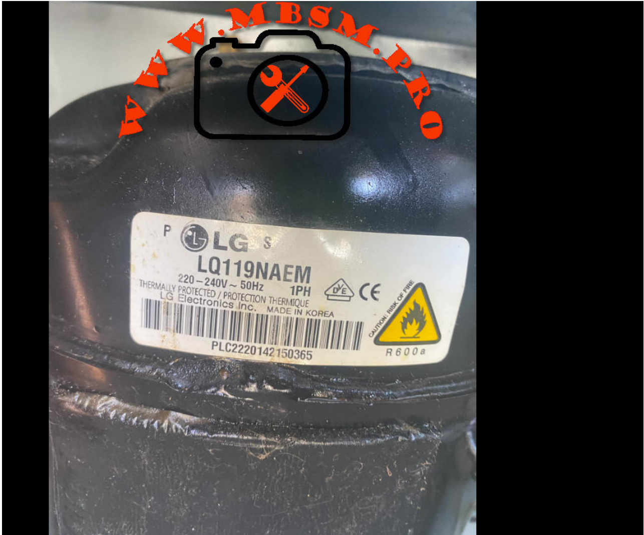
Mbsm.pro, Lg, compressor, LQ119NAEM, 1/3 hp, 227 w, lbp, 774 btu, r600a
