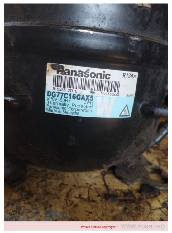
Mbsm.pro, Compressor, DG77C16GAX5,  $1/5\ hp++$ ,  $1/4\ hp-$ ,  $225\ w$ , Low Back Pressure, Refrigerant: R134a
