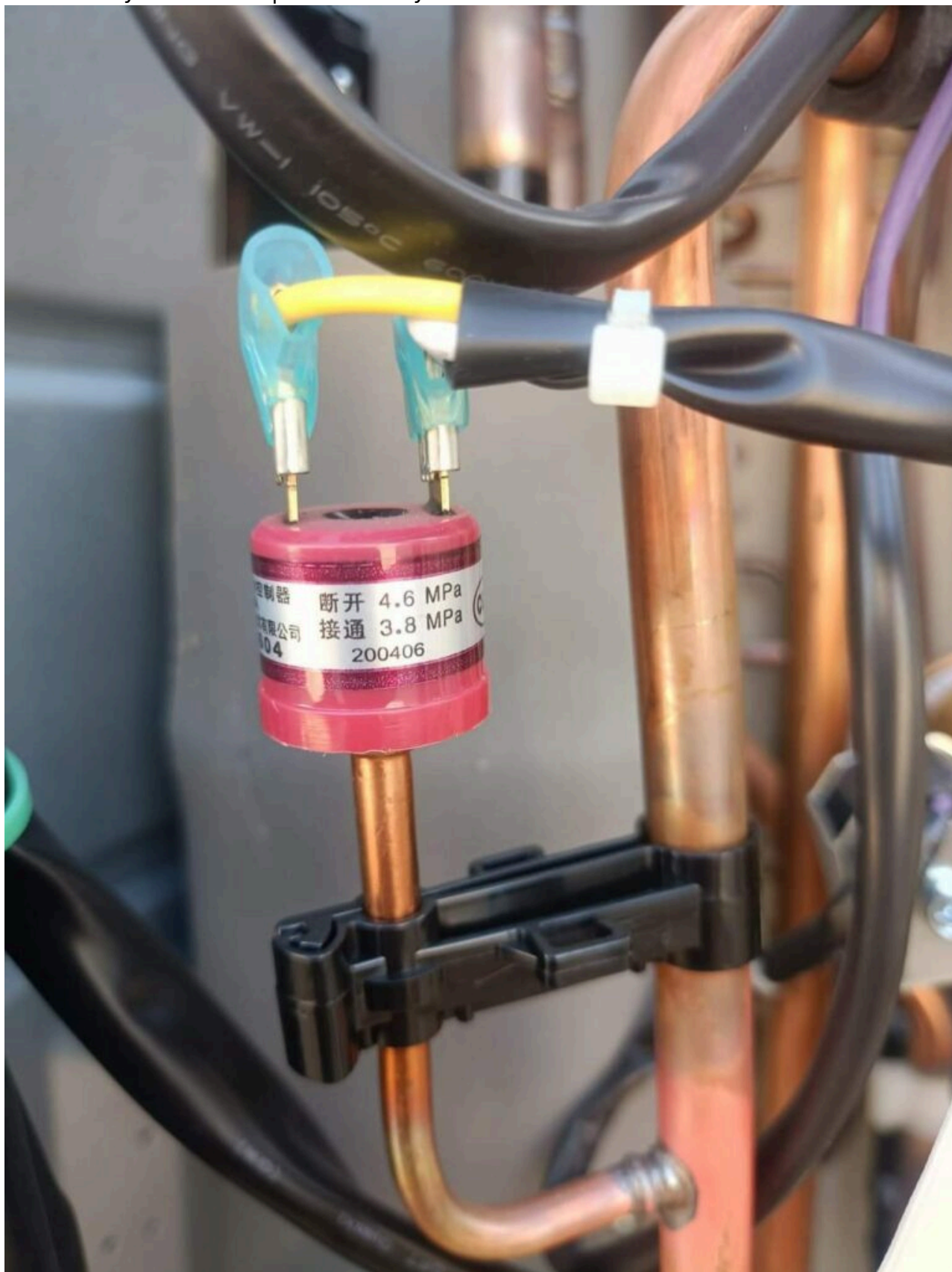
low-pressure cut-off switch
