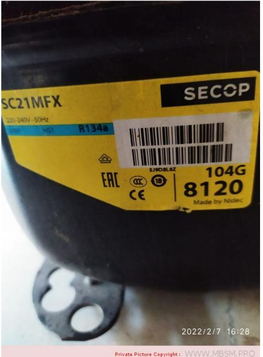
Mbsm.pro, Compressor, Danfoss, Secop, 5/8 hp++, SC21MFX, MBP, R134a, 220 V-240
