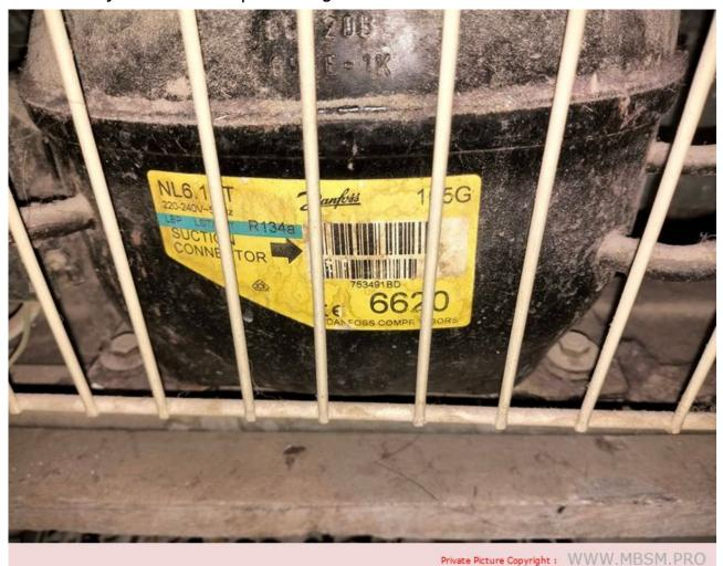
Mbsm.pro, Compressor, NL6.1FT, SECOP, 105G6620, DANFOSS, 1/6 hp, Lbp
