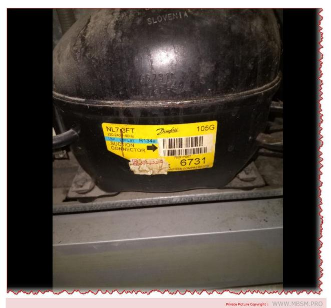
the 105G6731 is a model number for a tropical compressor manufactured by Secop, which is part of Danfoss. Here are the key specifications and details related to this compressor:
