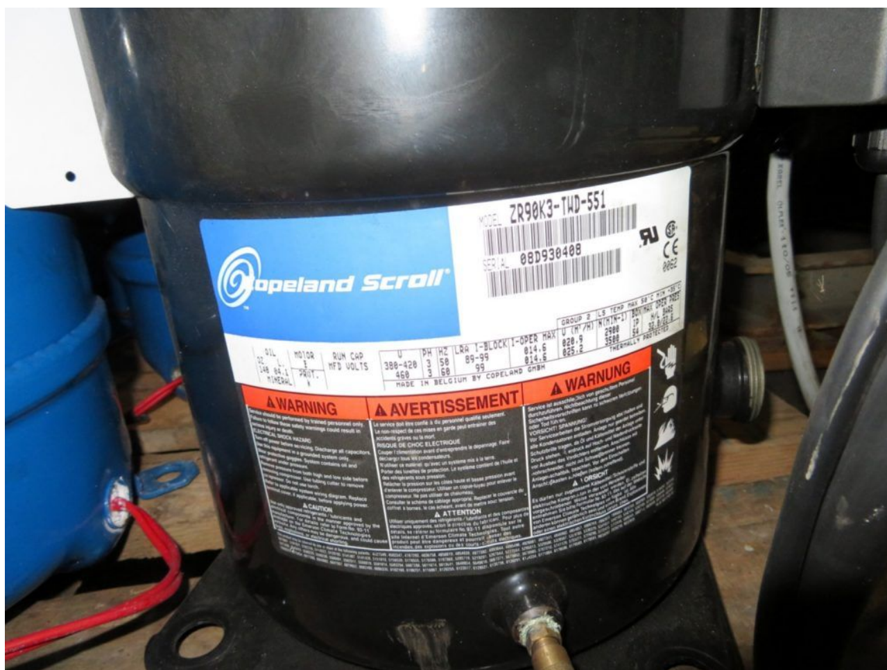
Mbsm.pro, Compressor, Copeland, ZR90K3-TWD-551, ZR90K3TWD551, 7.5 Hp, R22, 380-420/3/50Hz
