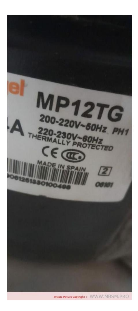
Mbsm.pro, COMPRESOR, SELLADO, 1/2 HP, 6269 BTU/h, R-404a, 220V, PH1, CSR, HMBP, CUBIGEL, MP12TG
