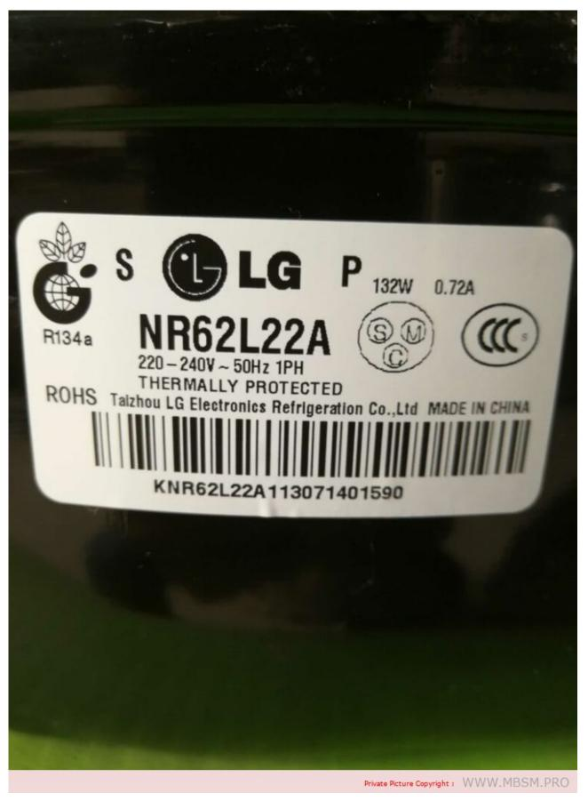
Mbsm.pro, Refrigerator, freezer, NR62L22A, 1/5 hp, Compressor, power, 132W, R134a
