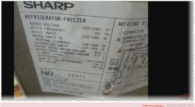
The Sharp refrigerator, with its low power consumption (170-190 watts), large storage capacity (577 liters), and eco-friendly refrigerant (HFC-134a), stands out as an excellent choice for households.
