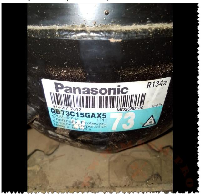
Mbsm.pro, Freezer, GR-EF40, TOSHIBA REFRIGERATOR-FREEZER, 335 L, Qb73c15gax5 ,R134a , Refrigeration Compressor ,1/4 Hp, Panasonic, QB series , 1Ph , 220V 50Hz Mbsm.pro, Compressor, ML52-1A, PN 2725, r12, QB66C13GAX5, 1/5 hp, r134a, freezer, 6 raks
