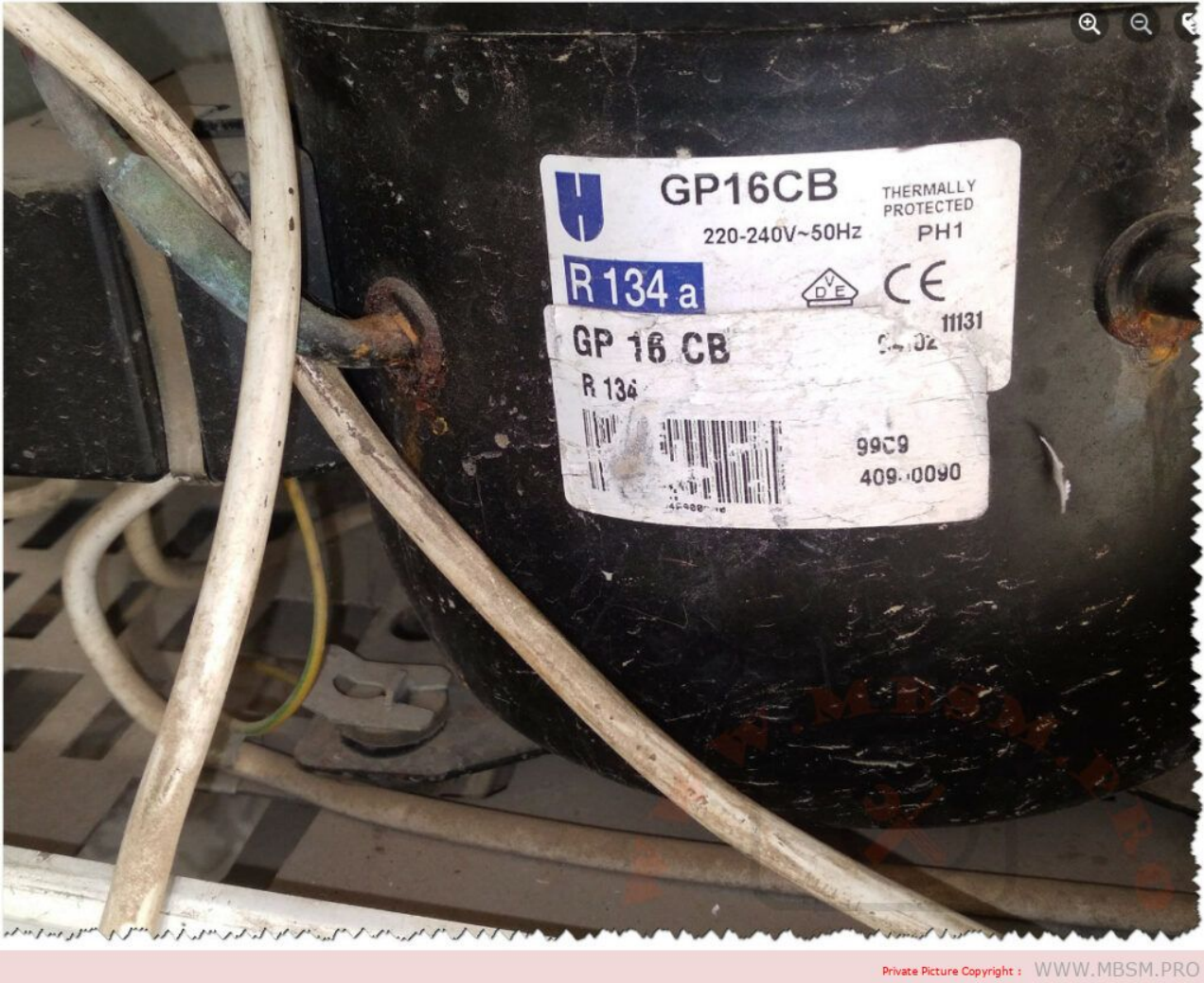
Mbsm.pro, Compressor, Cubigel, GP16CB, R134A, LBP, 3/8 hp
