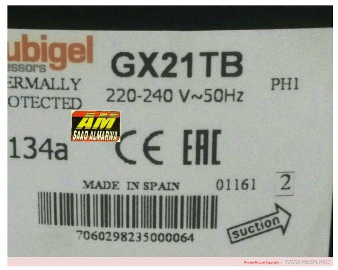
Mbsm.pro, Compressor, Cooling compressor Cubigel, GX21TB, 3/4 hp++, Hbp, 1 hp-, GPT18RA, 3/4 hp-, lbp, Country of origin Spain, r134a, 200-220/220-230V, 50/60Hz
