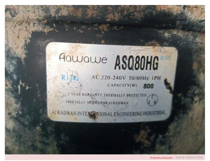
Mbsm.pro, Compressor, Huaguang, asq $80\,\mathrm{hg}$ , Q series,  $800\,\mathrm{w}$ , Hbp, r134a, 1/4 hp, cooling Aplication
