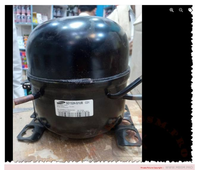
Mbsm.pro, R134A, 50Hz/ 60Hz, Samsung, Refrigerator, Compressor, SD152H, 1/6 hp, SD162H, 1/5 hp, 1bp
