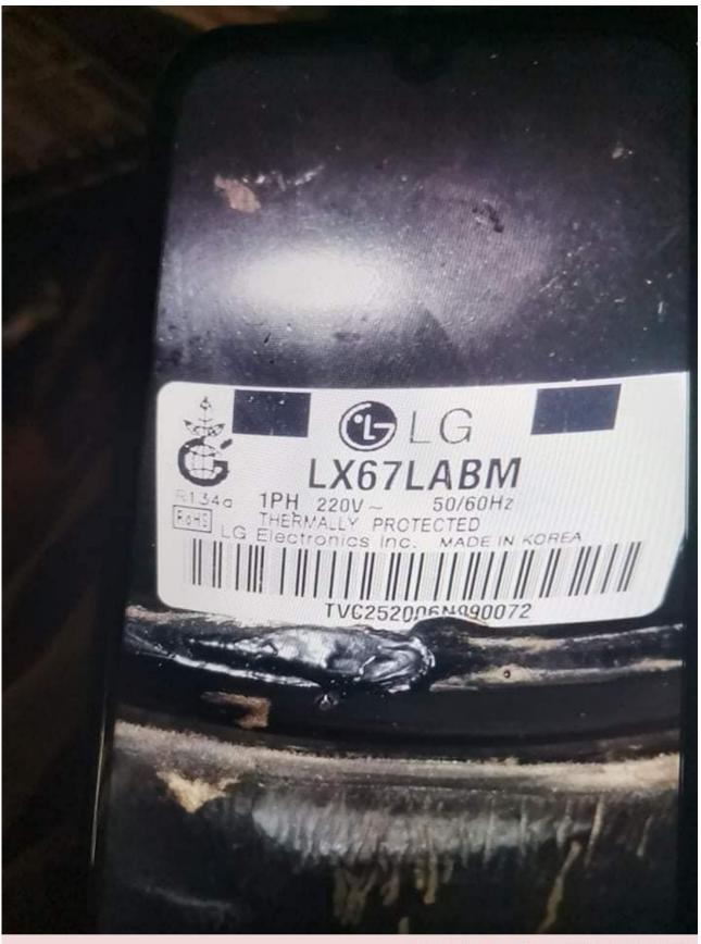
Mbsm.pro, Compressor, LG, LX67LABM, Refrigeration, 1/5 HP, LBP, RSCR, 180 W
