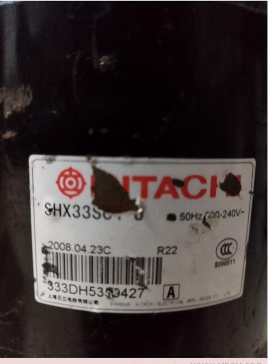
Private Picture Copyright: WWW.MBSM.PRO Mbsm.pro, compressor, Highly, hitachi, rotary, SHX33 , 2 hp, 17750 btu, R22
